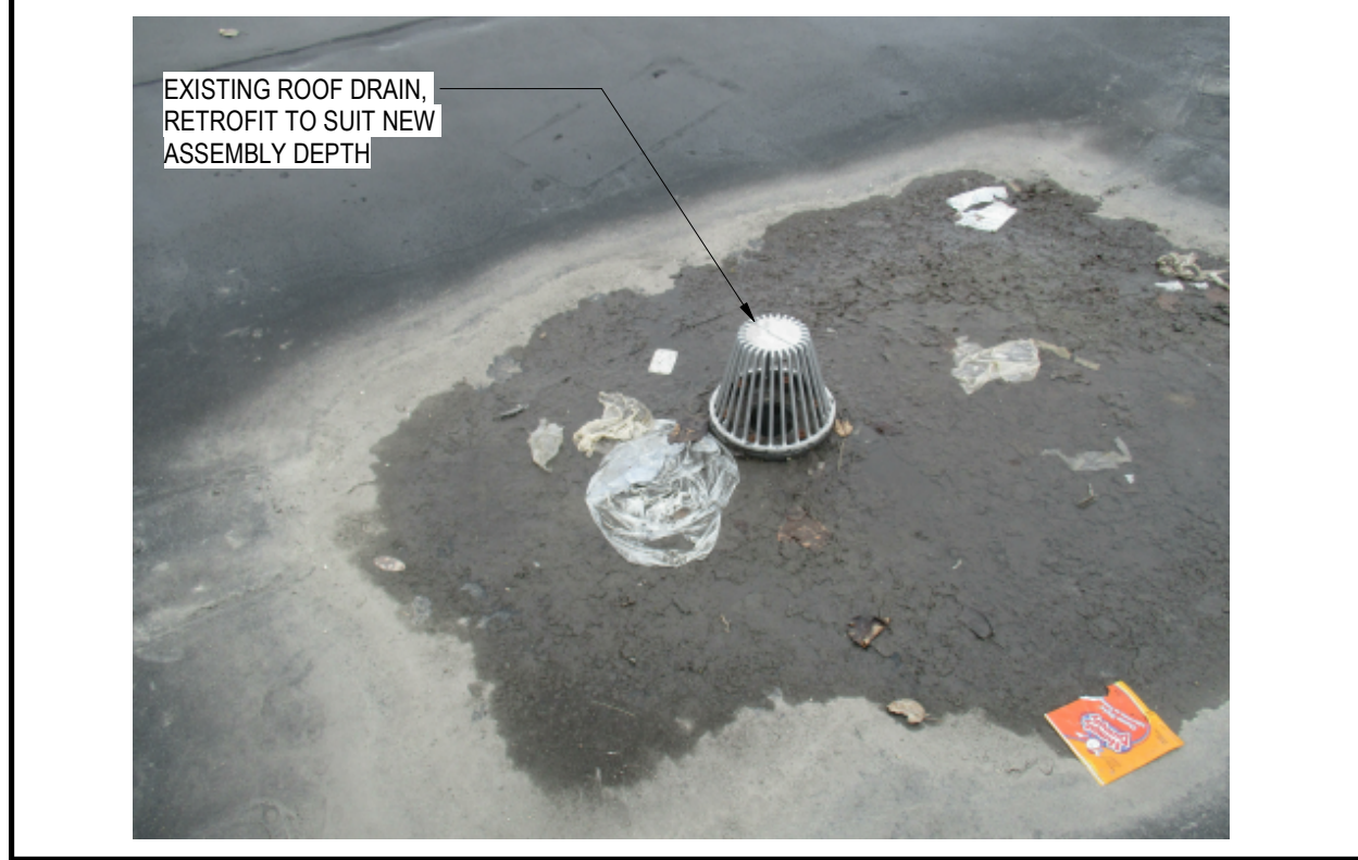
14 ROOF DRAIN A701 1:10
